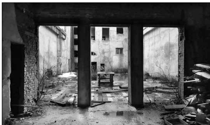
■ Foto 6. Locul restaurantului © VÁRADY Enikő, 2018 ■ Photo 6. Restaurant area © VÁRADY Enikő, 2018
