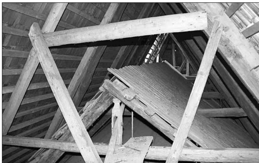
■ Foto. 3. Acoperișul secundar de peste naos, văzut dinspre altar © Laura ZAHARIA ■ Photo. 3. Secondary roof over the nave, view from the sanctuary © Laura ZAHARIA
